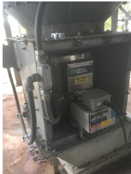
Figure 61 In-Line chute in a Zimmerman chute
